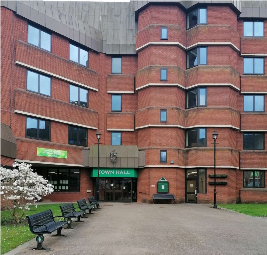
Figure 5: Redditch Town Hall
